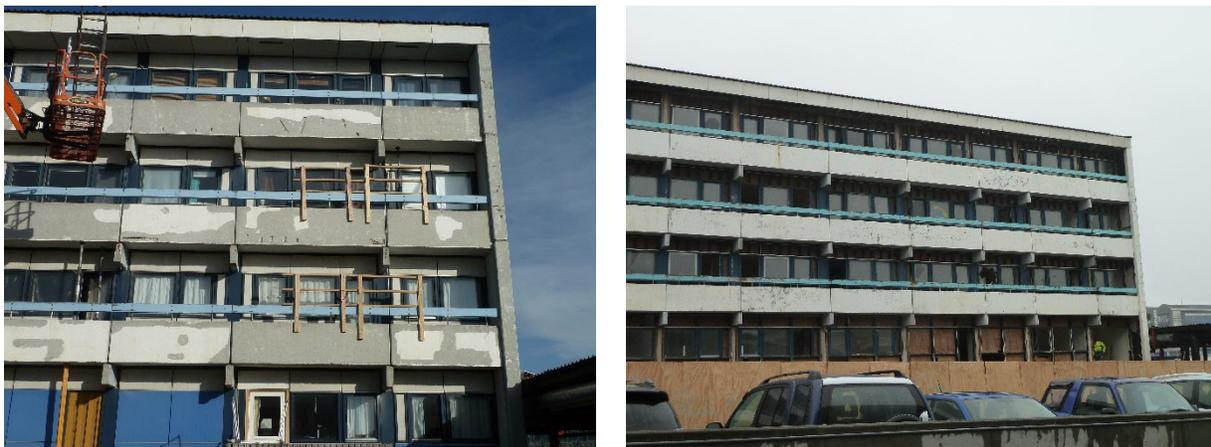
**FIGURE 1.** Illustration of the dilemma: The building block on the left is under refurbishment, while the building block on the right, from the same neighbourhood, is awaiting demolition. What technical and non-technical reasonings enable us to determine the real service life? On what basis was it decided to renovate the building on the left and not the one on the right?
