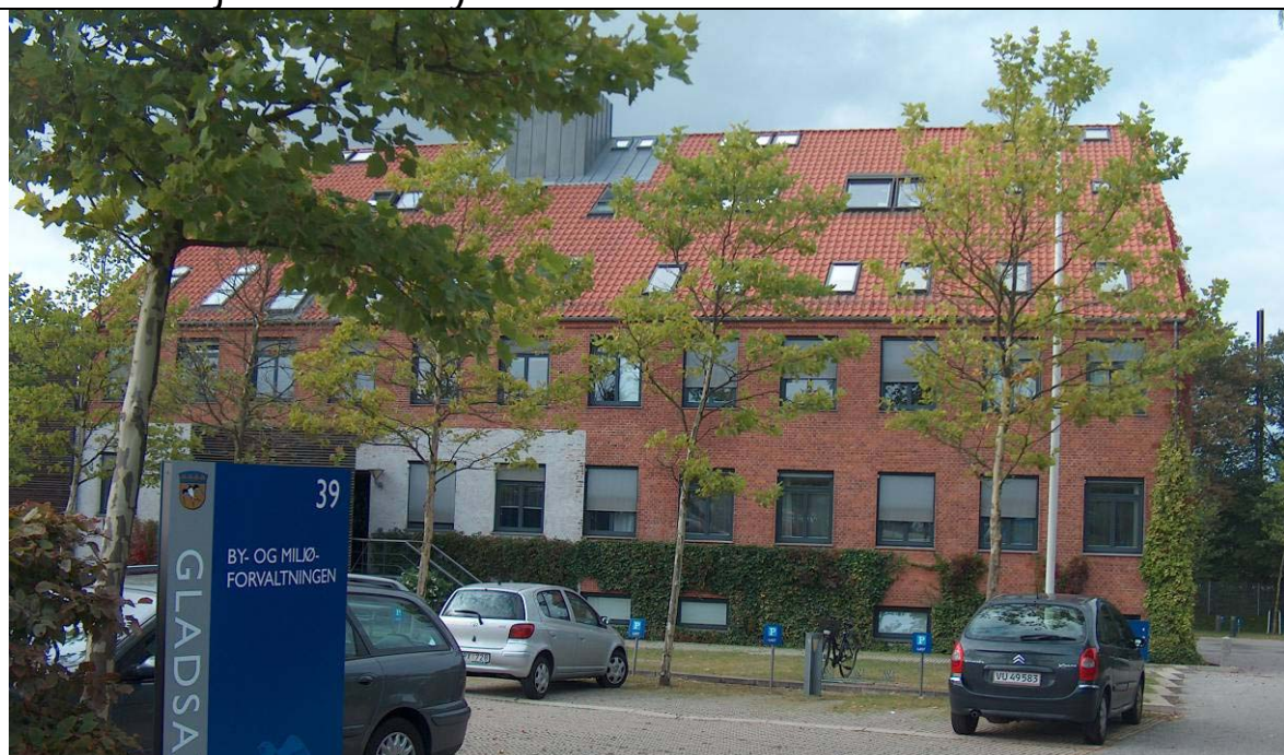
Rosenkæret 39, Office building, Gladsaxe Owner: private. User: Gladsaxe municipality.
