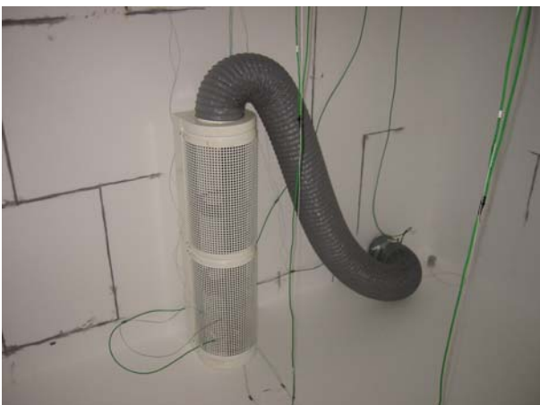
Figure 7. Inlet device for displacement ventilation.
