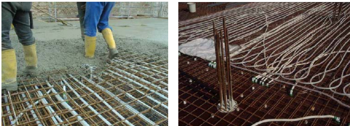
Figure 3.4 – Concrete lying on the reinforcement grid with attached pipes (Hauser 2005)
