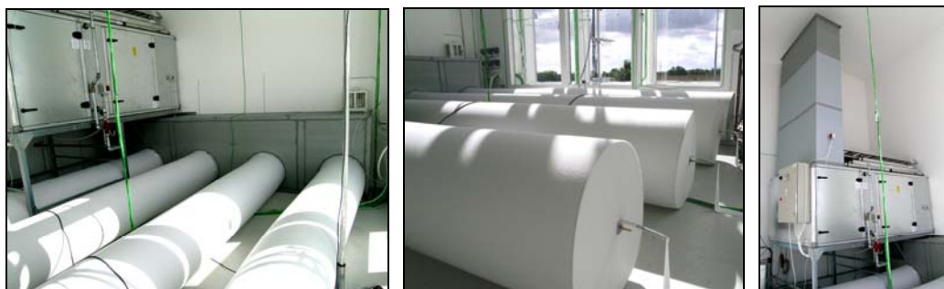
Figure 3. KE-low impulse fabric ducts in the experiment room (left, centre), Ventilation system in the experiment room (right).
