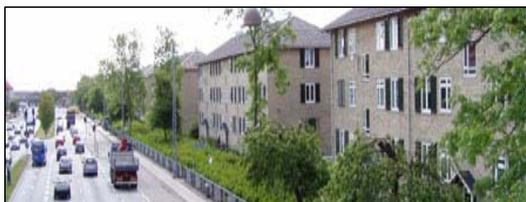
Figure 5 – The required window sound insulation is calculated based on the facade requirement and the performance and areas of components.
