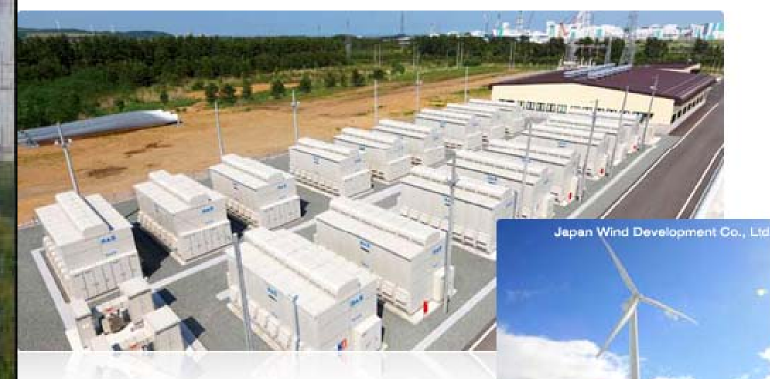
34MW NAS storage, Japan
