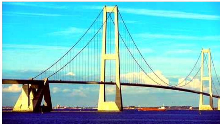
Figure 3. Great Belt East Bridge, Denmark (taken from Huynh [1]).
