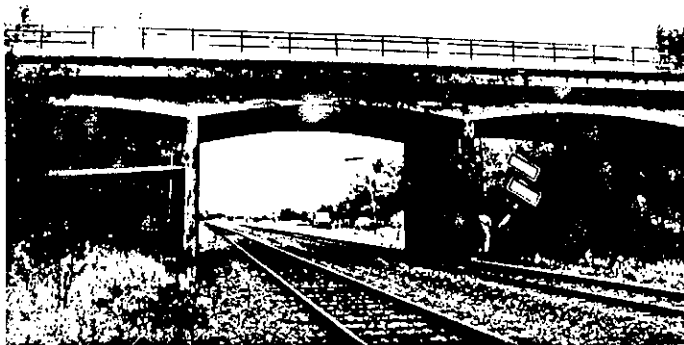
Figure 1. Front of Bridge.
