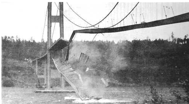
Figure 1. Tacoma Narrows Bridge Collapse (1940)
