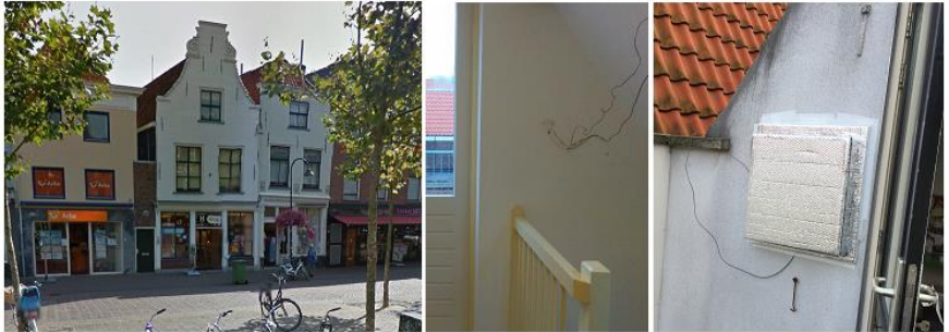
Fig. 2 Case study - The whole building (left), the inside surface of the wall (middle), and the outside surface and sensors covered by the box (right). Delft, Nov 2014
