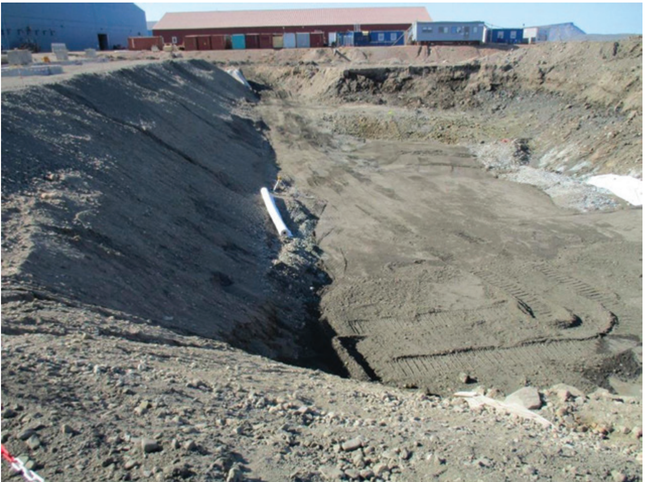
Figure 10.19 Over-excavation for construction of slab-on-grade structure, Thule Air Base (photo by Kevin Bjella).
