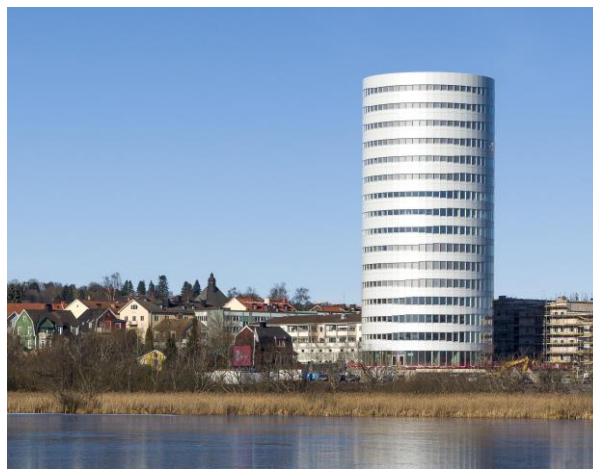
Figure 3 Munksjötornet building in Jönköping (Sweden)
