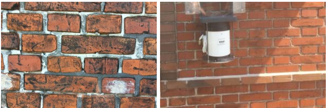
Figure 6: Masonry on façades of test building 1 (left) and test building 2 (right)
