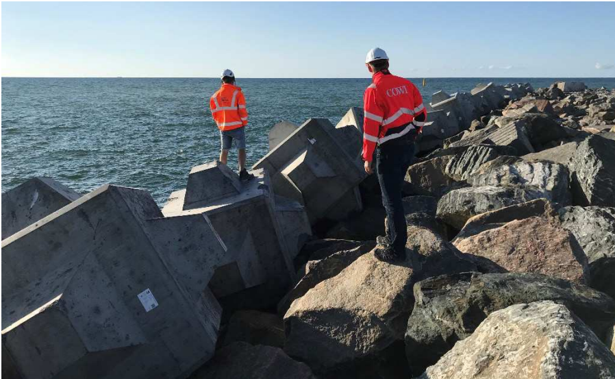
Fig. 2. Cubipod ® armour unit placed on the new breakwater in Hansthalm (summer 2018).
