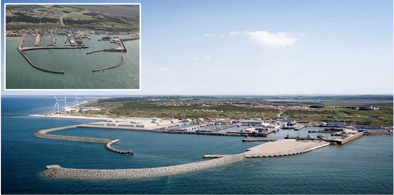
Fig. 1. Existing port layout (top right) and new port expansion (illustration by Per Aarsleff A/S).
