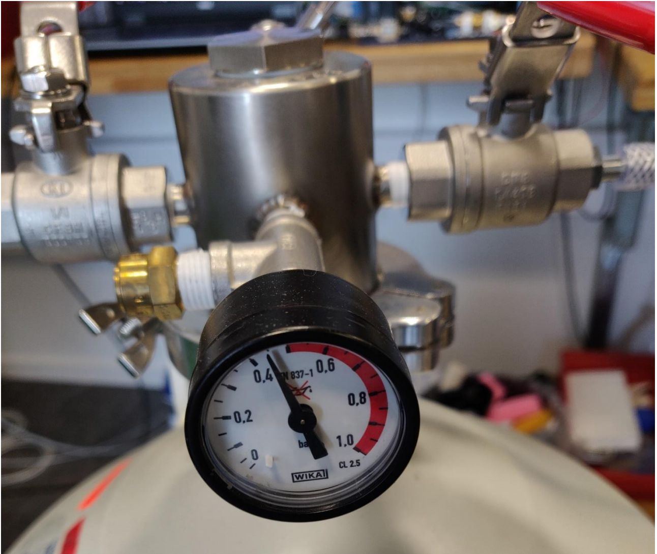
Figure 8: Adequate pressure for the liquid nitrogen storage dewar.
