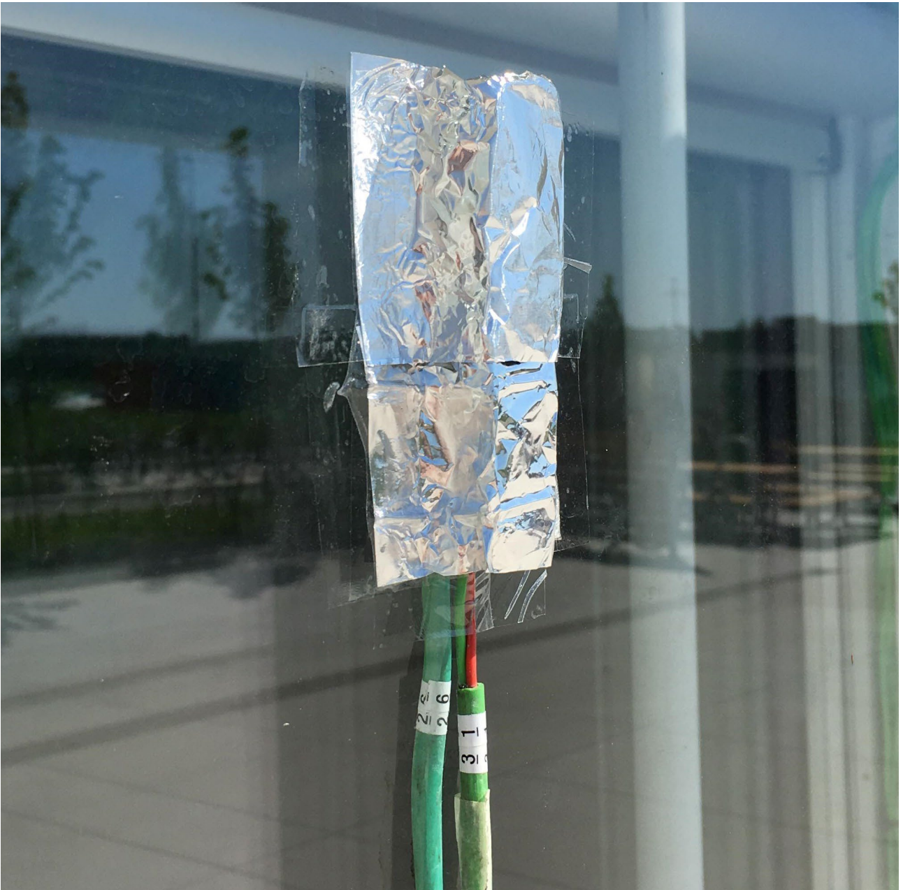
Figure 28: Thick type-K thermocouples for surface temperature measurements in the DSF 23 setup [1].
