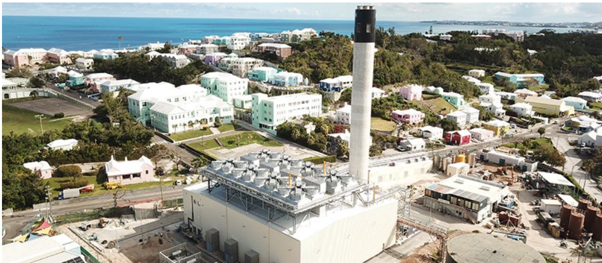
Figure 4 – BWSC's North Power Station project in Bermuda 2 .
