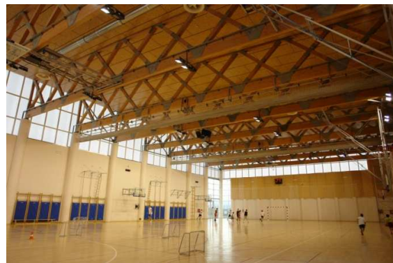
Figure 4: Timber truss structure of the sport hall in Samobor
