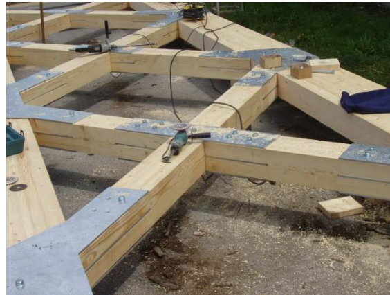
Figure 3: Details of tensile and compressive elements
