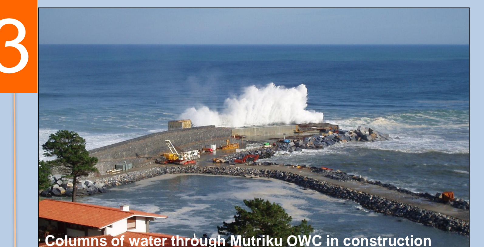
Columns of water through Mutriku OWC in construction
