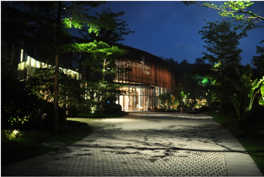
Figure 3: Crescent Hills, a large hot spring resort, located in Zhangzhou, Fujian. Carry Yu completed the lighting design of this hotel in 2015 [4]
