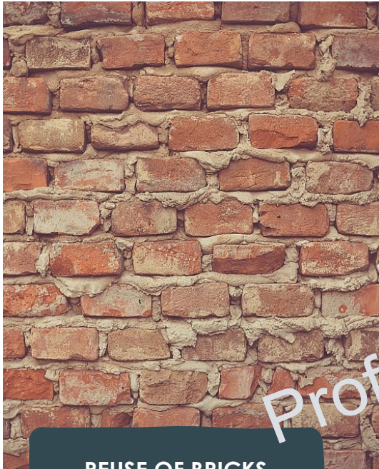
REUSE OF BRICKS
