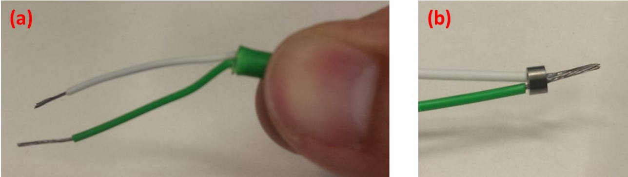
Figure 8: (a) remove plastic insulation; (b) place the pressure connector.
