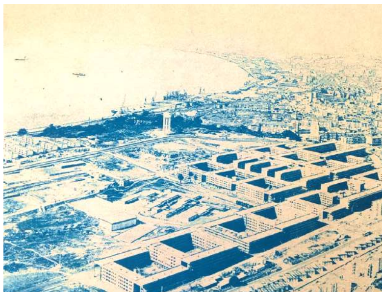
Fig.1 – Bela Vista Neighbourhood under construction. Source: Silva, 1988
