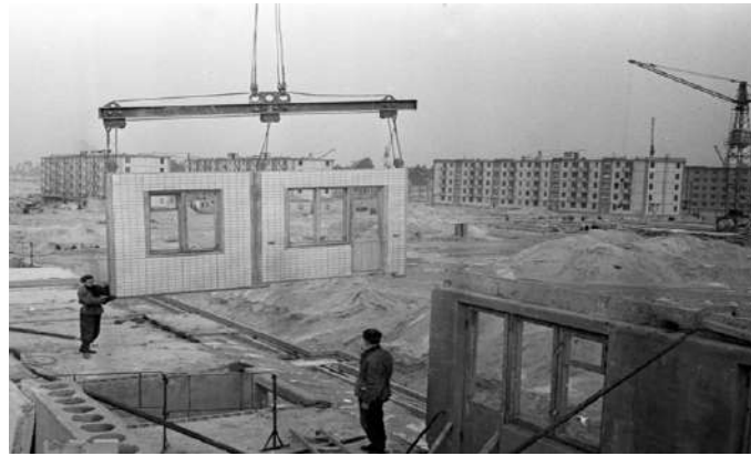
Fig.3 – Prefabricated panel construction. Source: TsDKFFA of Ukraine
