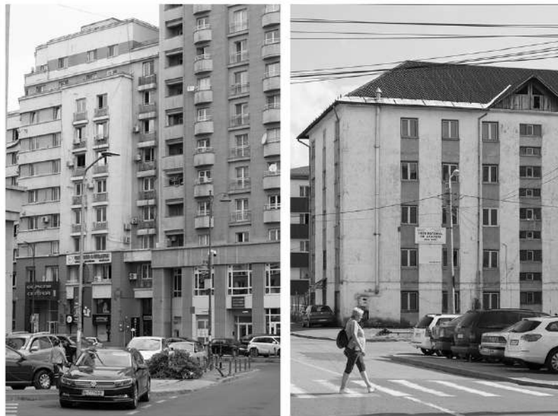
Fig. 3 – Left – Bucharest building; Right – Baia Mare building. Source: personal photographs.
