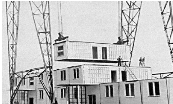
Fig.4 – Mounting volumetric blocks. Source: Ataev. 1967. Technology and Economics of Volume-Block House Construction
