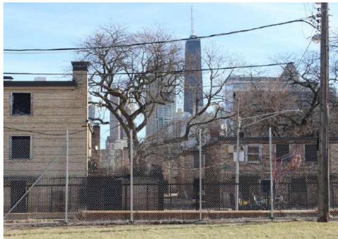
Fig.2 – More than two-third of the row-houses composed of 440 family flats were evacuated by 2012 and they are still waiting for private investors who are interested in their renovation. Source: Author's own, 2020.
