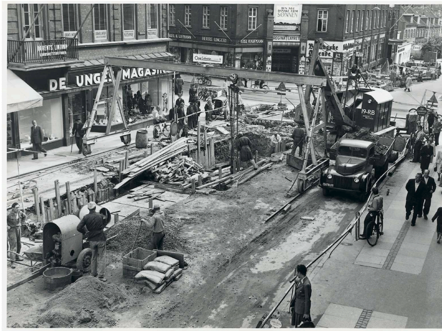
Fig. 2. District heating construction works, Aarhus. Picture source: Affaldvarme Aarhus. Reprinted with permission.
