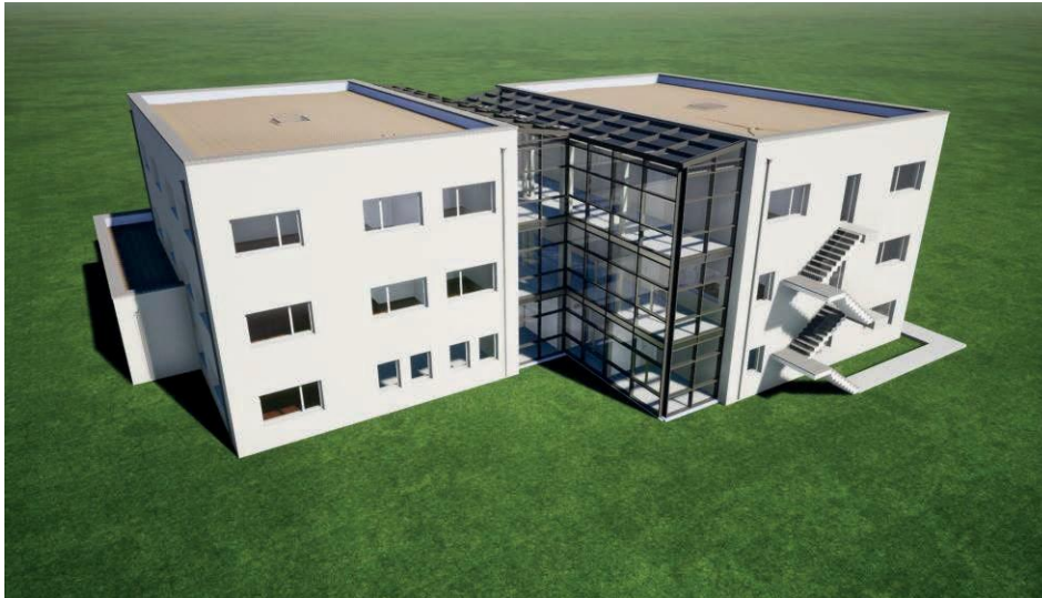
Figure 1: Completed building as a result of the module (HTWK Leipzig: left part, TU Dresden: right part)
