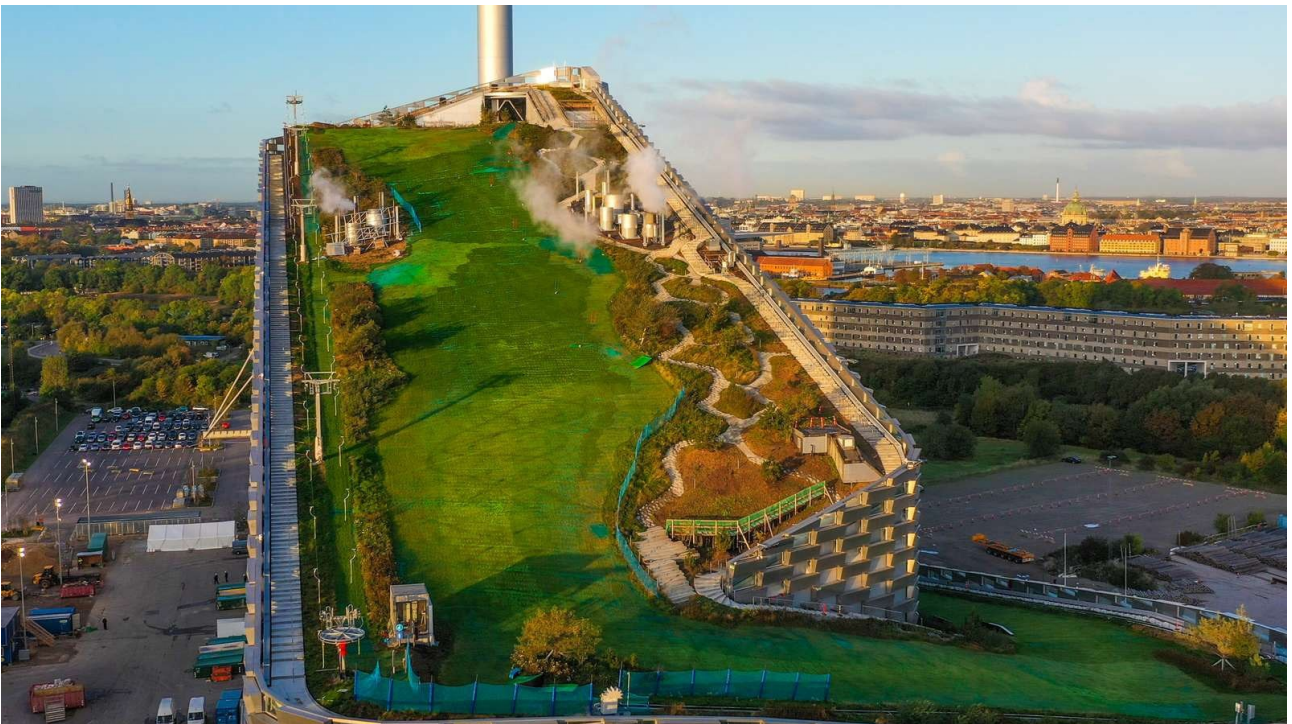
Figure 8. Combined heat and power waste-to-Energy plant, CopenHill. Copenhill is also an outdoor recreational facility with an artificial ski-slope and other outdoor activities on the roof. Copenhill opened in 2017. Credits: Press/CopenHill.
