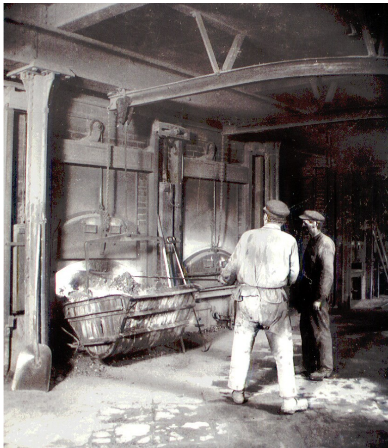
Figure 3. The incineration plant. 1903. Printed with permission from Frederiksberg Forsyning.
