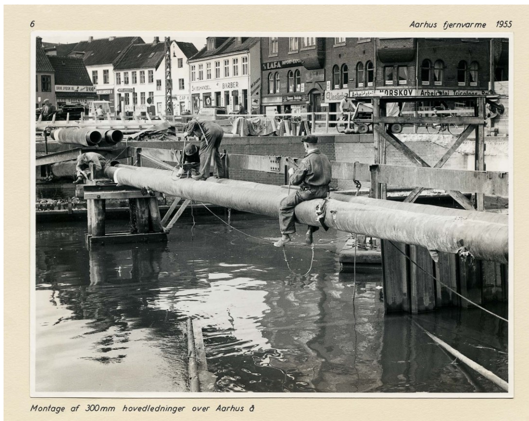
Figure 5: Installing 300 mm main pipes across Aarhus Creek, 1955. Printed with permission from Affaldvarme Århus
