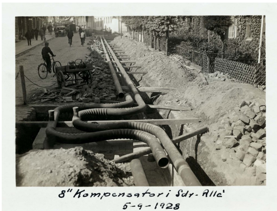
Figure 4: Compensator in Søndre Allé, Århus, Denmark. 1928. Printed with permission from Affaldvarme Århus.
