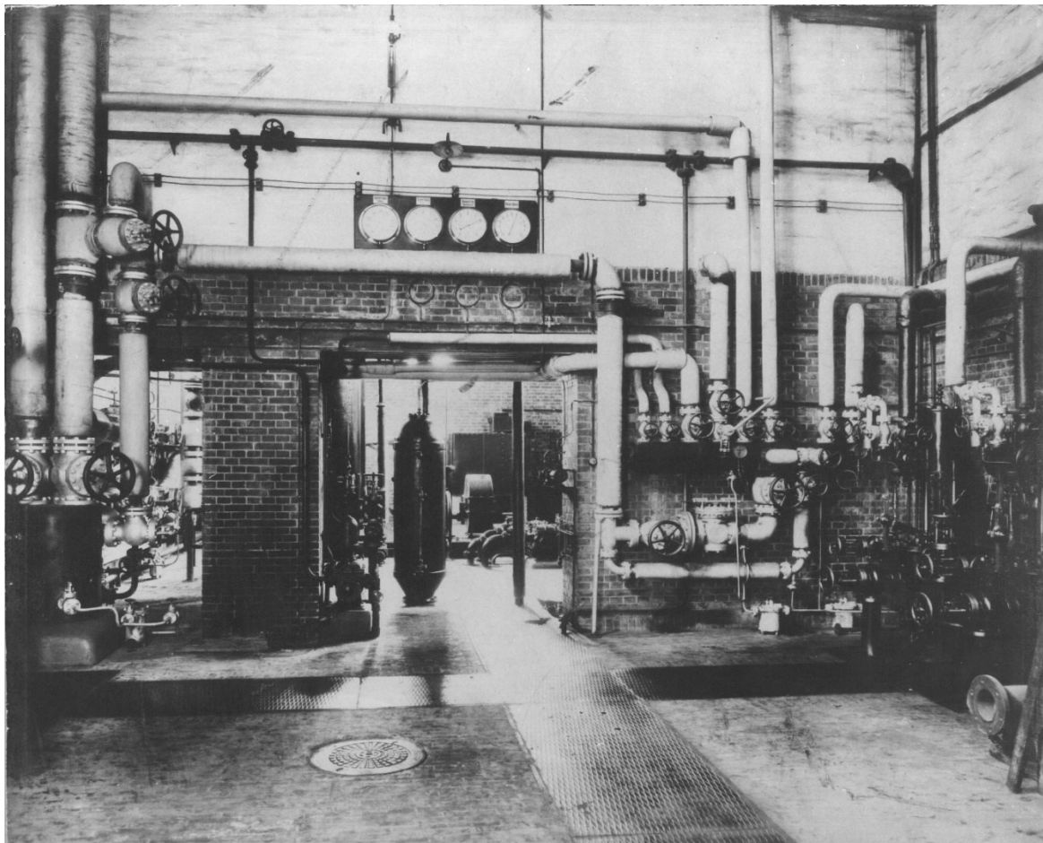
Figure 1. The incineration plant. 1903. Printed with permission from Frederiksberg Forsyning.
