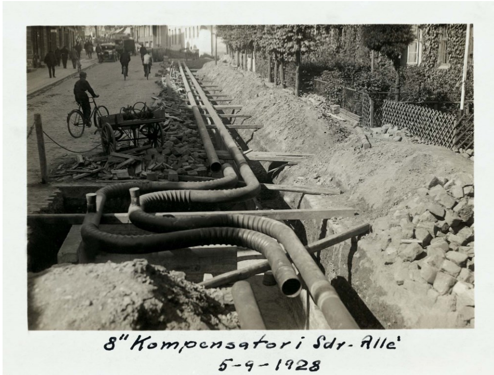
Figure 4: Compensator in Søndre Allé, Århus, Denmark. 1928. Printed with permission from Affaldvarme Århus.
