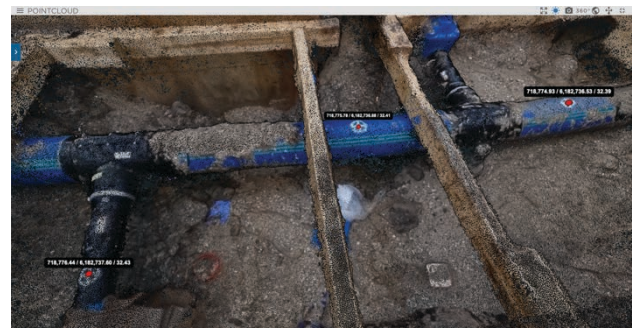
Figure 4. Check Points (CPs) marked as white crosses, which coordinates has been identified in the point cloud.
