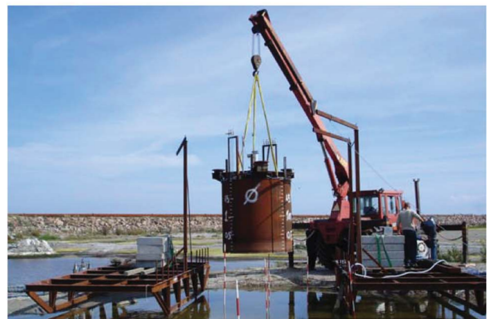
Fig. 4. (a) Location of the experimental medium-scale model of a monobucket foundation in Frederikshavn (map data ©2021 Google); and (b) bucket foundation used in the offshore tests performed (image by Lars Bo Ibsen).
