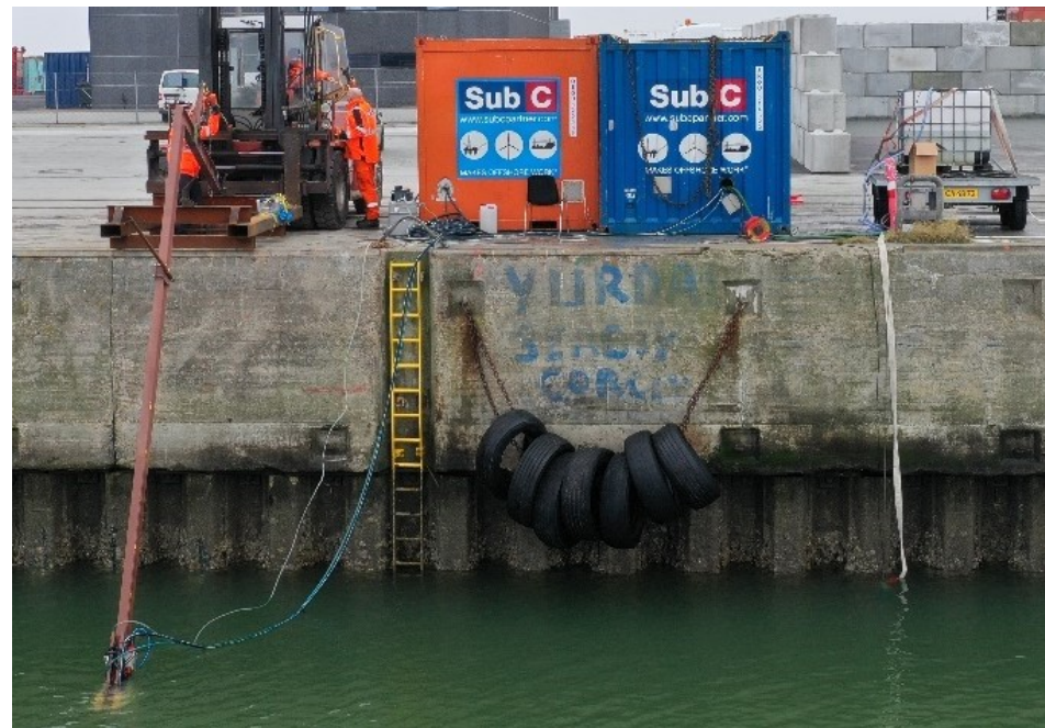
Figure 4. Test setup for cleaning test at Port of Esbjerg.
