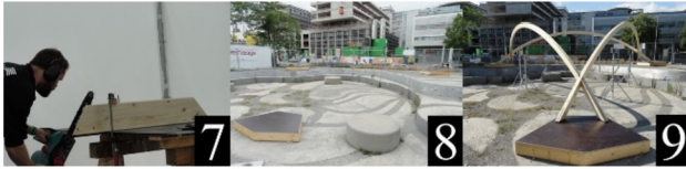
Figure 2: Fabrication and positioning of timber beams (Source: © BioMat at ITKE/University of Stuttgart).
