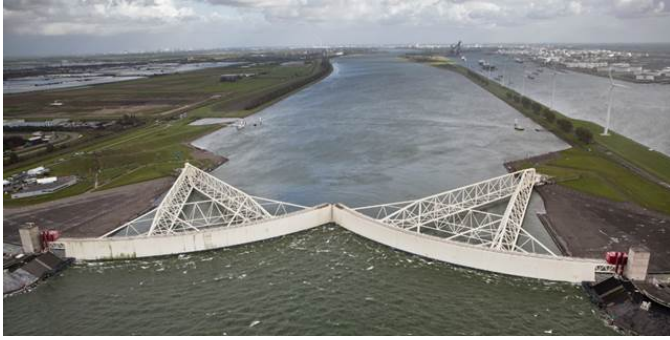
Fig. 1. The Maeslantkering in its closed position. Image from https://beeldbank.rws.nl , Rijkswaterstaat.
