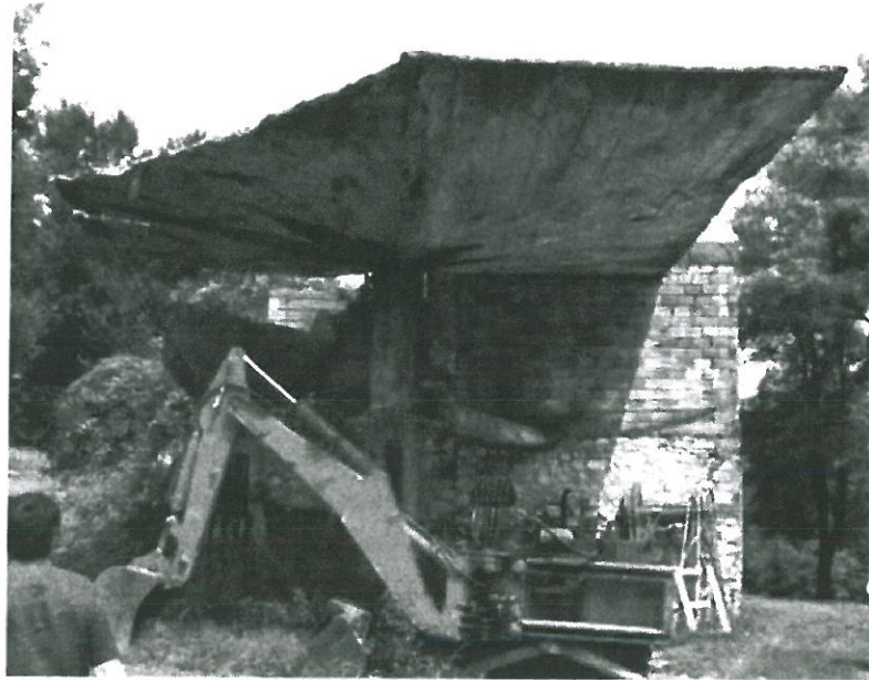
Fig. 6. Umbrella Structure, Zandobbio, Bergamo (1959-60)
