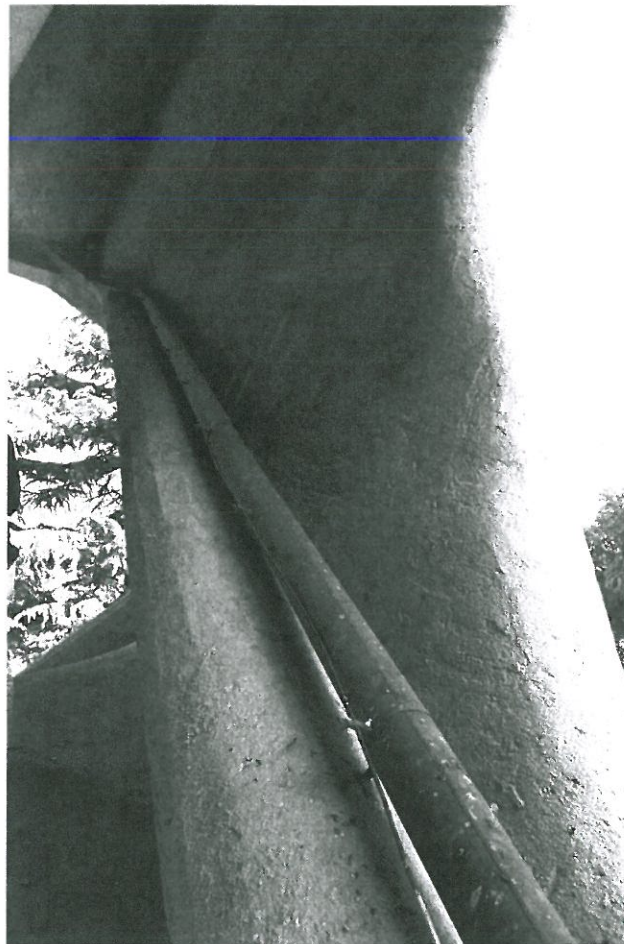
Fig. 30. Gutter pipes hidden in the structure.
