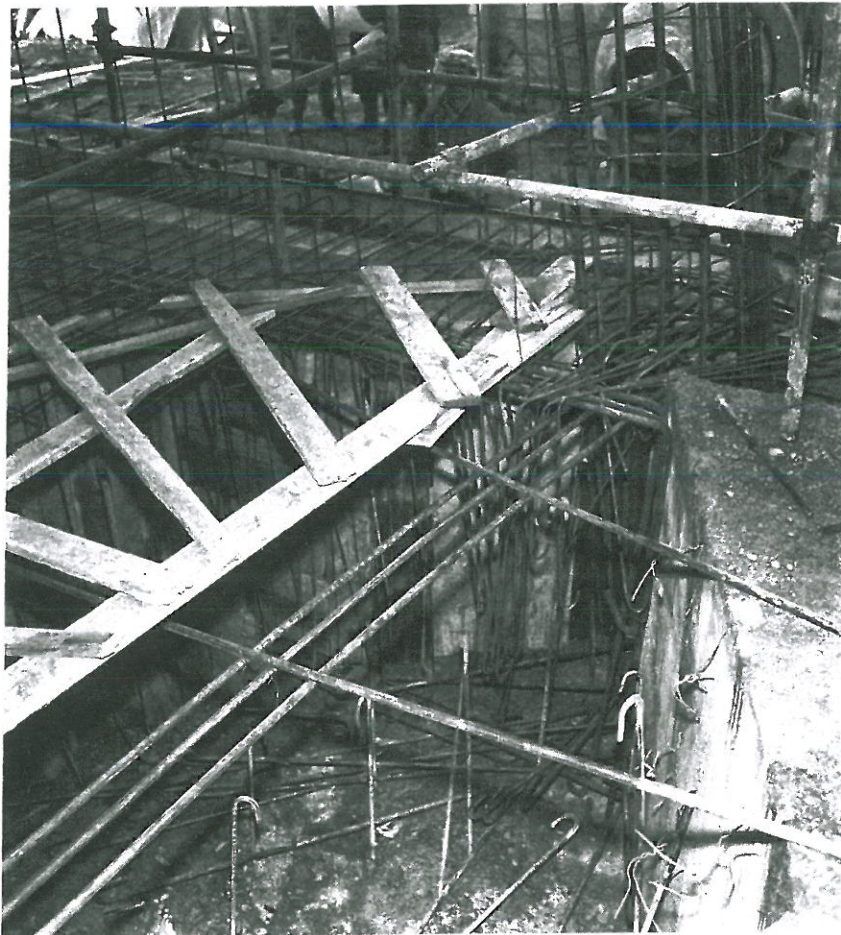
Fig. 25. Casting of the foundation beams.
