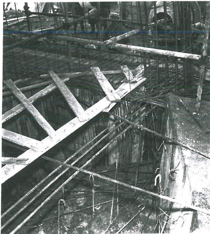
Fig. 25. Casting of the foundation beams.
