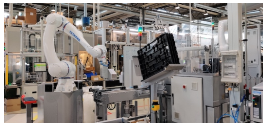
(b) The pick-and-place cobot at company B. It picks the products from the transportation boxes and places them on the conveyor belt to be transported to the next step in the assembly line.
