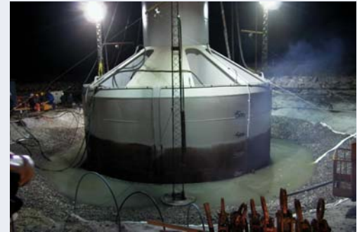
The monopod bucket foundation is installed using suction assisted penetration Frederikshavn 2002
