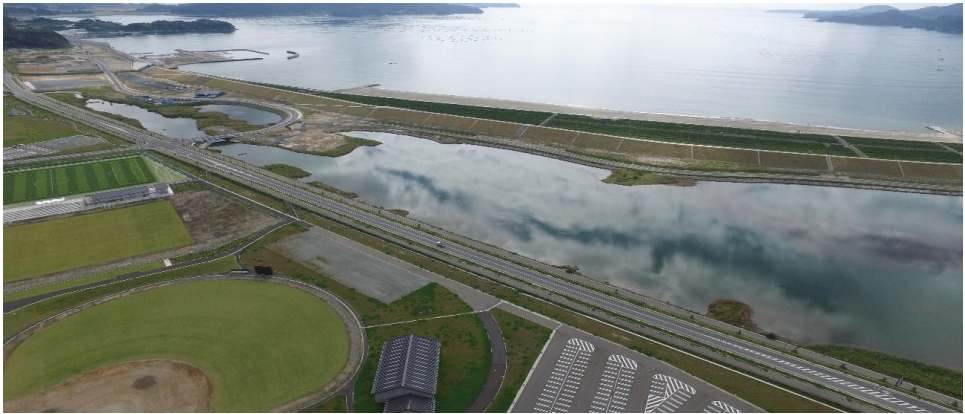
Photo of Furukawanuma Marsh; the tidal salt marsh is surrounded by the construction of a 12.5-meter-high and a 2-km-long seawall.
