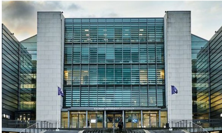
The control of the indoor environment in a modern office building in Copenhagen, Denmark
