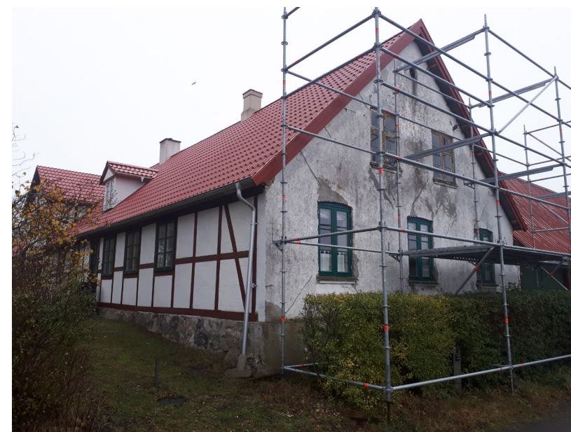
Byhus i Utterslev under renovering
