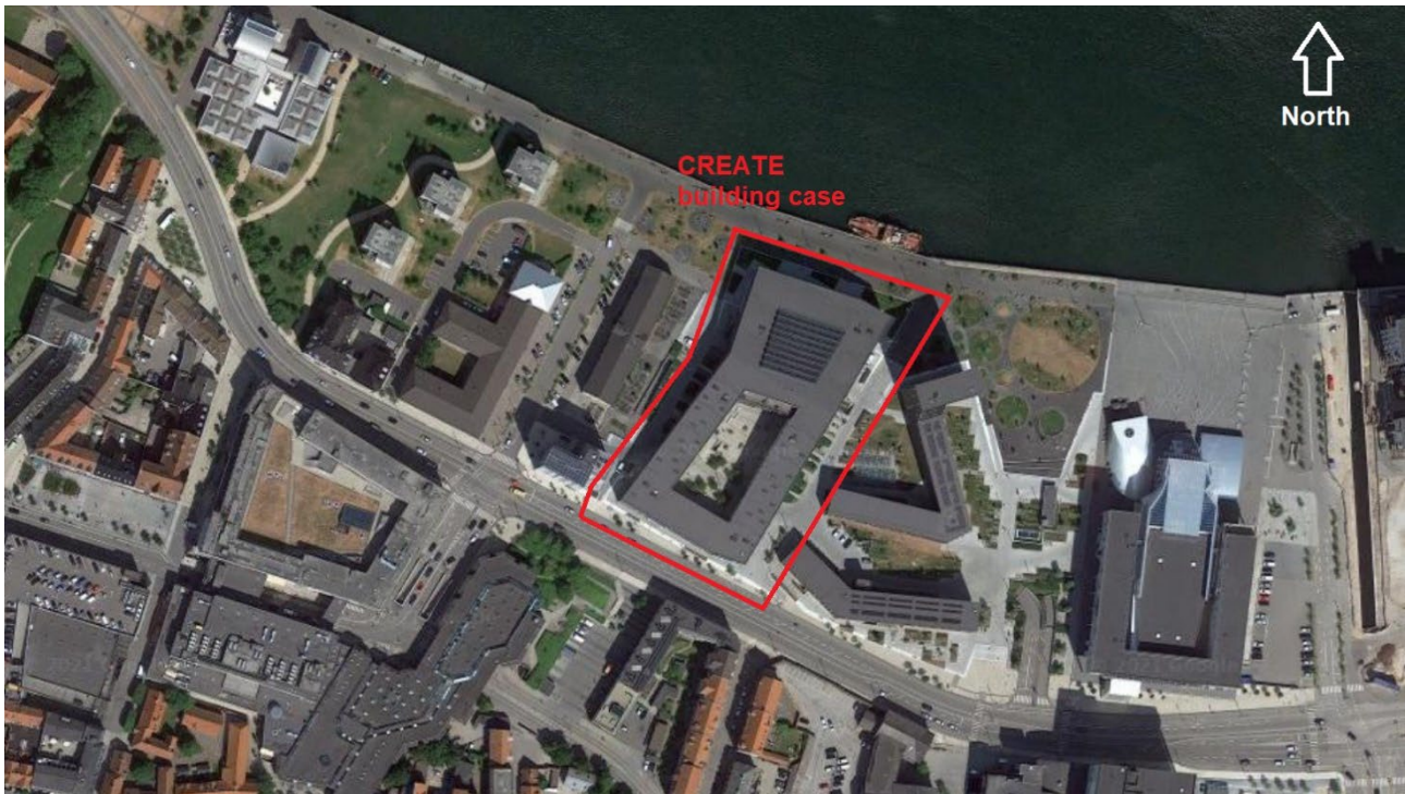
Figure 4: Aerial view of the CREATE building in its surrounding environment in Aalborg city center.
