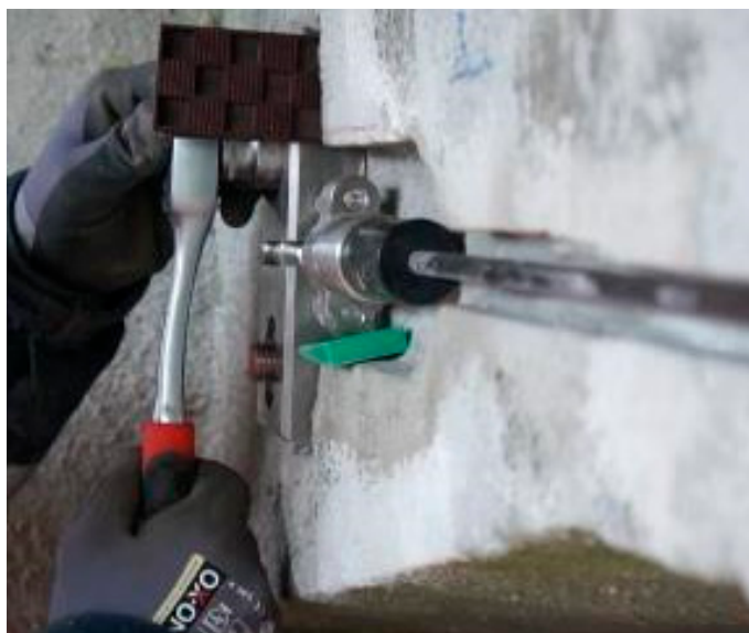
Figure 10. Installation of the through going threaded bars. Photograph by S&P.
