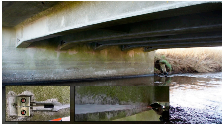
Figure 17. The final result of the applied strengthening. Photograph by S&P.
