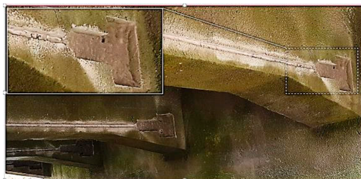
Figure 9. Cut grooves used for the strengthening system mounting. Photograph by S&P.
