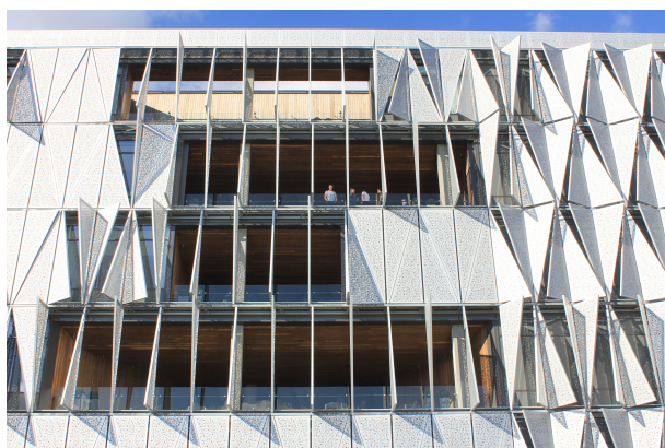
Figure 1. University of South Denmark, responsive facade with moving mechanical parts.
