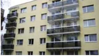
Major renovation of an apartment building in Tallinn: before and after
