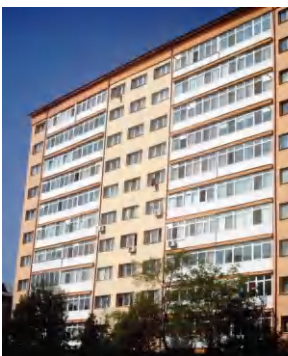
Rehabilitated block of flats
