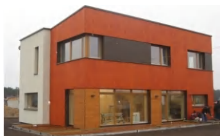
The construction site of the first passive house
