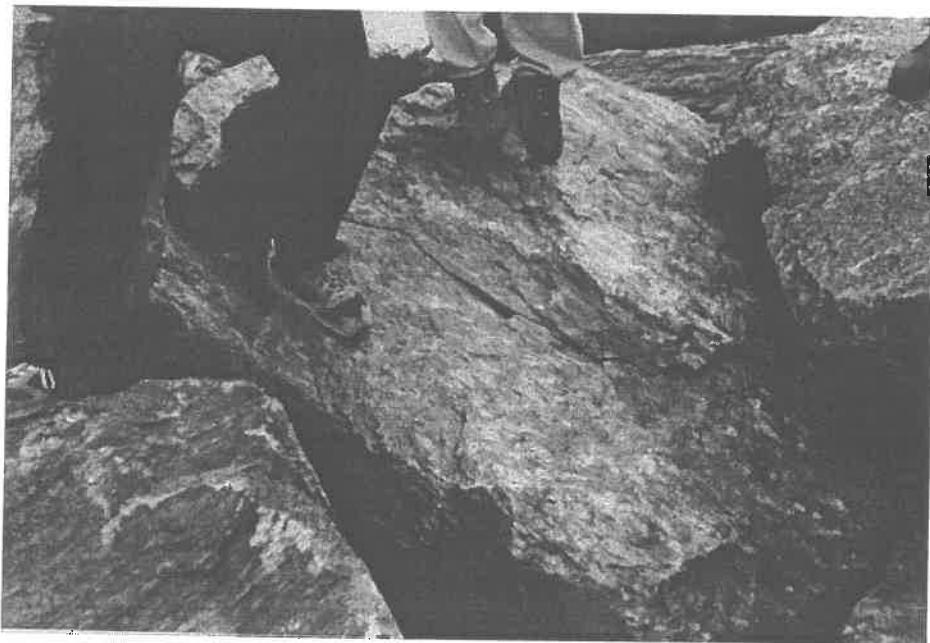
Photo from Norwegian berm breakwater
