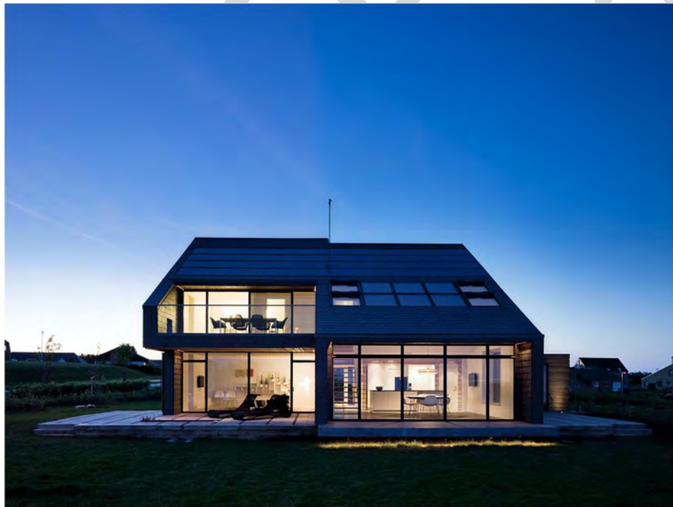
Fig. 1. Home for Life: the south-facing smart window facade, the roof with integrated roof top windows, solar cells, solar heat panels, and the weather station on top of the roof. Photo by Adam Mørk.
