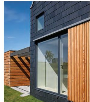
THE EXTERIOR: Solar panels that produce electricity, solar collectors that capture heat, and skylights vie for space on the house's Scandinavian-style slanted roof. The facades and roof were built out of wood and slate, which require less energy to produce than other commonly used materials.
