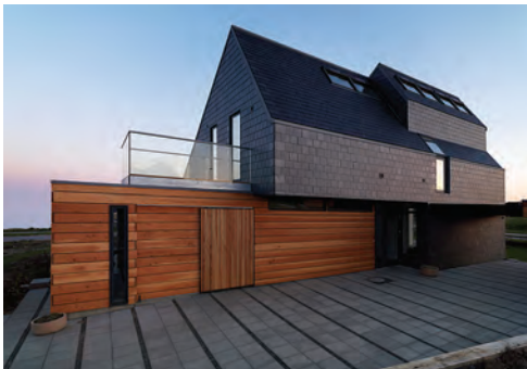
THE EXTERIOR: Solar panels that produce electricity, solar collectors that capture heat, and skylights vie for space on the house's Scandinavian-style slanted roof. The facades and roof were built out of wood and slate, which require less energy to produce than other commonly used materials.
