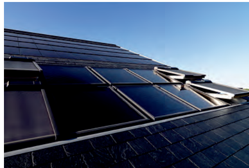
THE EXTERIOR: Solar panels that produce electricity, solar collectors that capture heat, and skylights vie for space on the house's Scandinavian-style slanted roof. The facades and roof were built out of wood and slate, which require less energy to produce than other commonly used materials.
