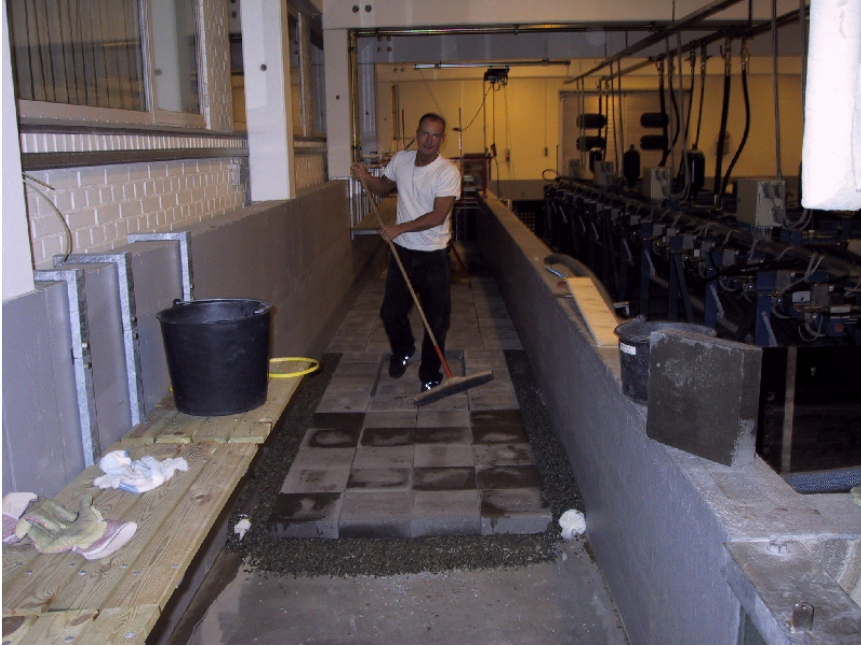
Figure 19: Construction of the 'reef' in the wave flume.
