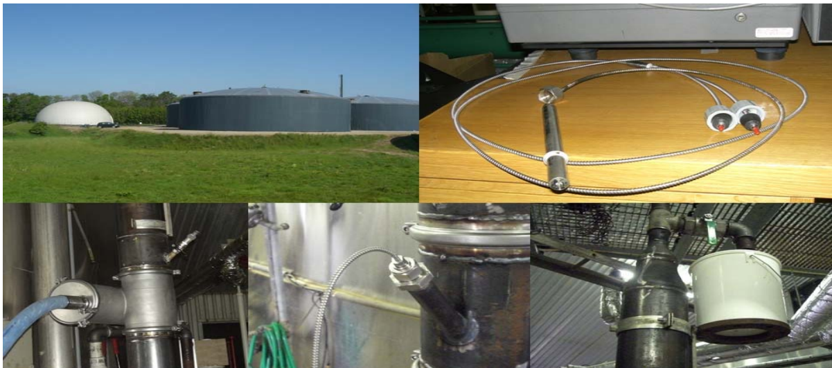
Fig. 7.1: Full scale PAT studies managed during 2007. Trials and tests were conducted at LinkoGas a.m.b.a., Rødding, Denmark. PAT tools for on-line monitoring facilities were mounted at a recurrent loop integrated with fermentor no. 3 volume 2400 m 3 . Testing of various NIR probes of transflexive and reflexion types was conducted. Lower right photo shows the sampling point for chemical reference analysis.
