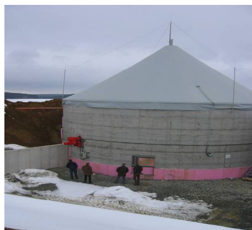
Figure 2. Fermenter No. 2 at Strem biogas plant. Insulation was not completed because this mesophilic fermentation process generated a surplus of heat surpassing that needed for keeping the process temperature constant. Inoculum at this biogas plant was cow manure but, after start-up, the feedstock was almost exclusively maize silage. Photo JBHN, 03/05-2005.
