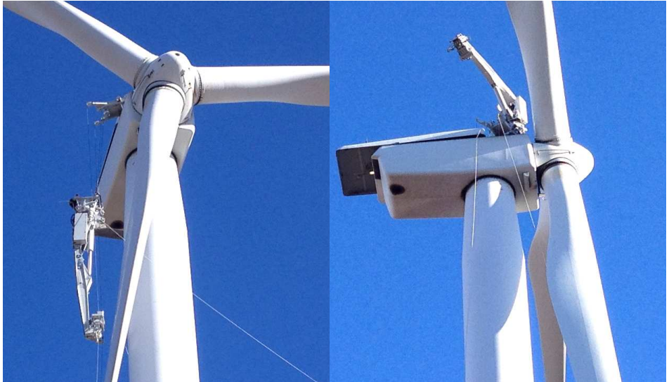
Figure 1.3: A potential motor application is as yaw motor at Liftras self hoisting cranes. Here one is during installation and after the installation on the top of the nacelle of a wind Turbine.
