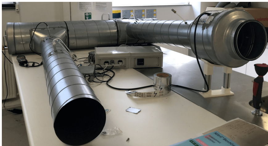
Figure 5-11 Partial experimental setup. Reactor and side ducts, fan module and power box.
