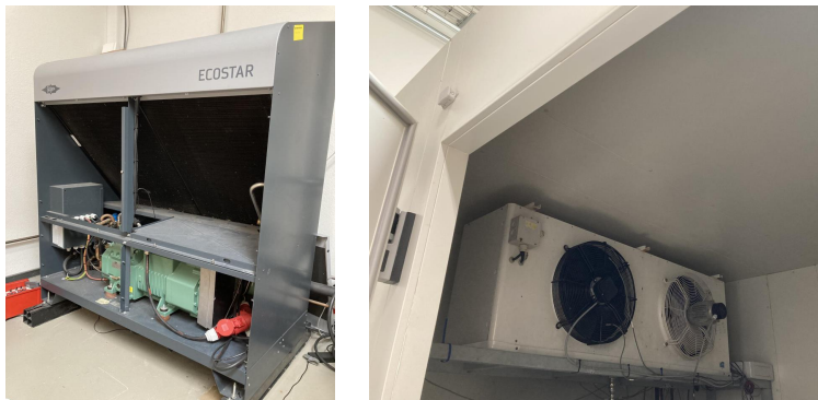
Fig. 4: Condensing unit of the laboratory setup at left and the evaporation side which is inside of the cold room at right. This setup is used for data collection in Papers A and B.
