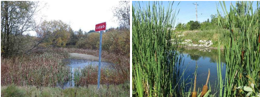
Picture 1-1 Stormwater retention ponds. The picture on the left illustrates a pond in Denmark (Jutland), while the one on the right shows a pond in Canada (Peterborough) with several inlet pipes.
